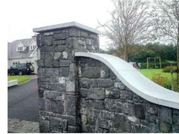
GRANITE STONE WALLS.
